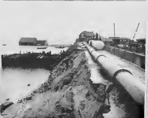
THE RAGING NORTH SEA cut a path of destruction through the Lowlands the strength of Holland's dykes could stem the flow. This view shows a break in the ancient town of Zierikzee where over 155 million cubic meters flooded. NOORDZEE RABIOSO a habri un camina di destruccion over di Holanda. Na a taken di dikan di North Sea por a wata e calamidad. E vista aki ta muestra mensa den coracian di e antiguo pueblo Zierikzee unda mas cu 155 mion cubic meters inundate e polder.
